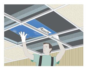
Next, drop the SkyTile into the Elevator.
